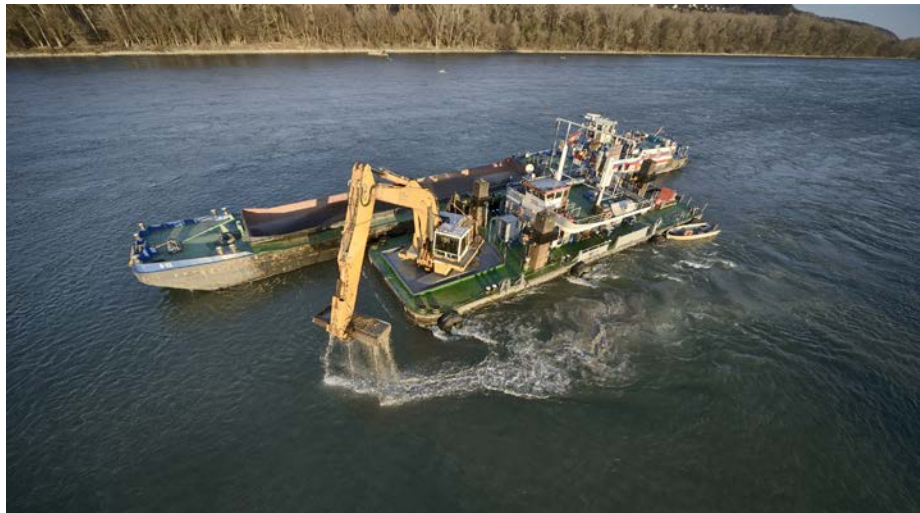
Dredging works with backhoe dredger in combination with hopper barges on the free-flowing section between Vienna and Bratislava
