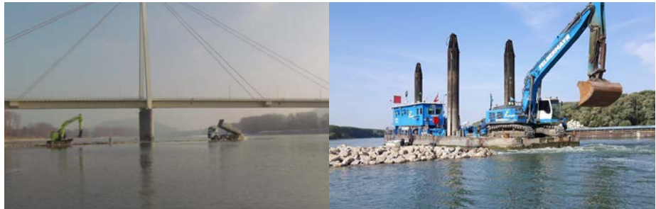
Hydraulic engineering optimisation on the Austrian Danube: Extension of current groynes near Bad Deutsch-Altenburg and Treuschütt on the free-flowing section between Vienna and Bratislava
