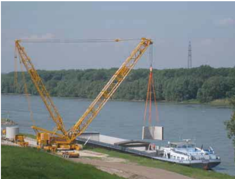
Mobile crane with caterpillar track system
