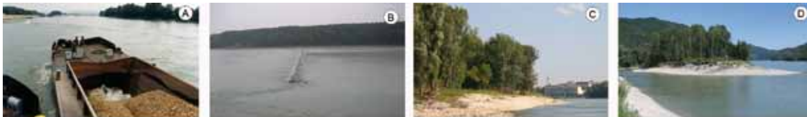
Riverbed adjustment and granulometric riverbed improvement – testing the method of placing
