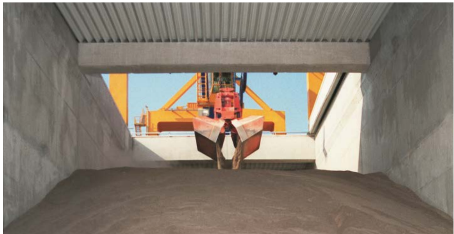
Bulk goods storage
